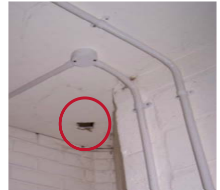
Viewing Hole into Bunker
