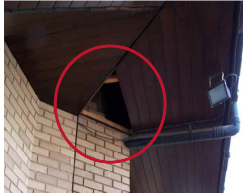
Access Point to Ceiling Void
